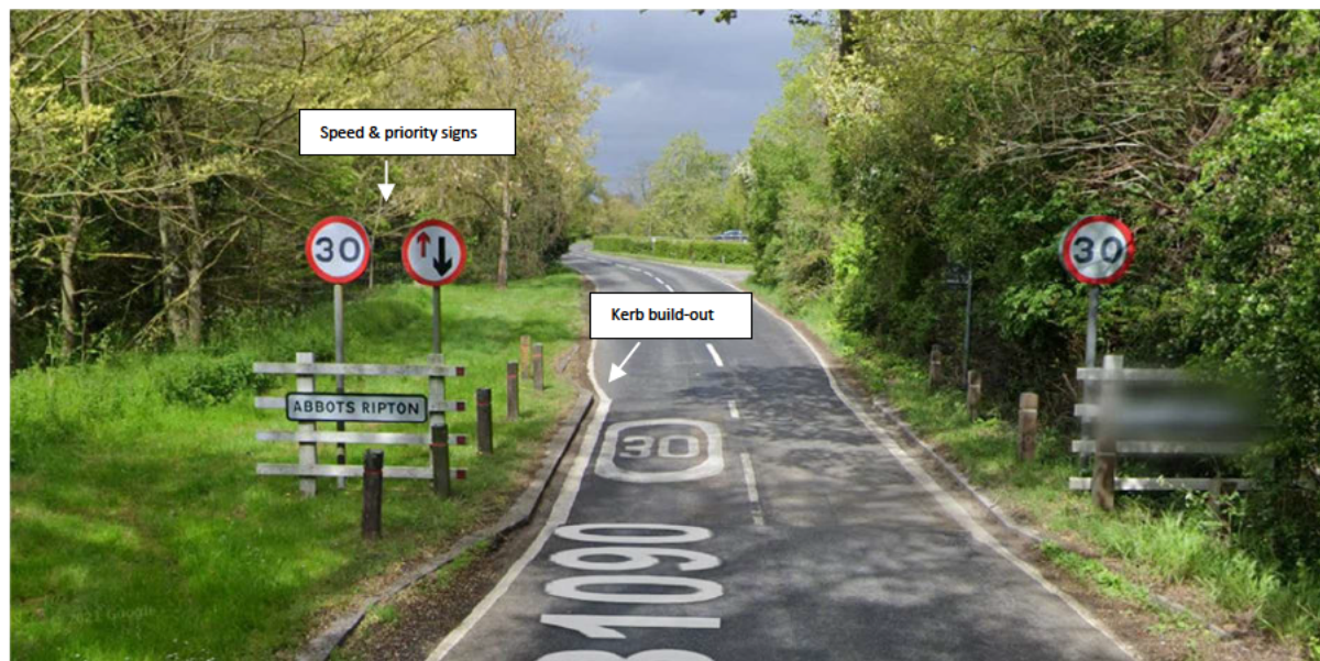
Figure 13: An example where a kerb build out has been used to cause a slight reduction in carriageway width
